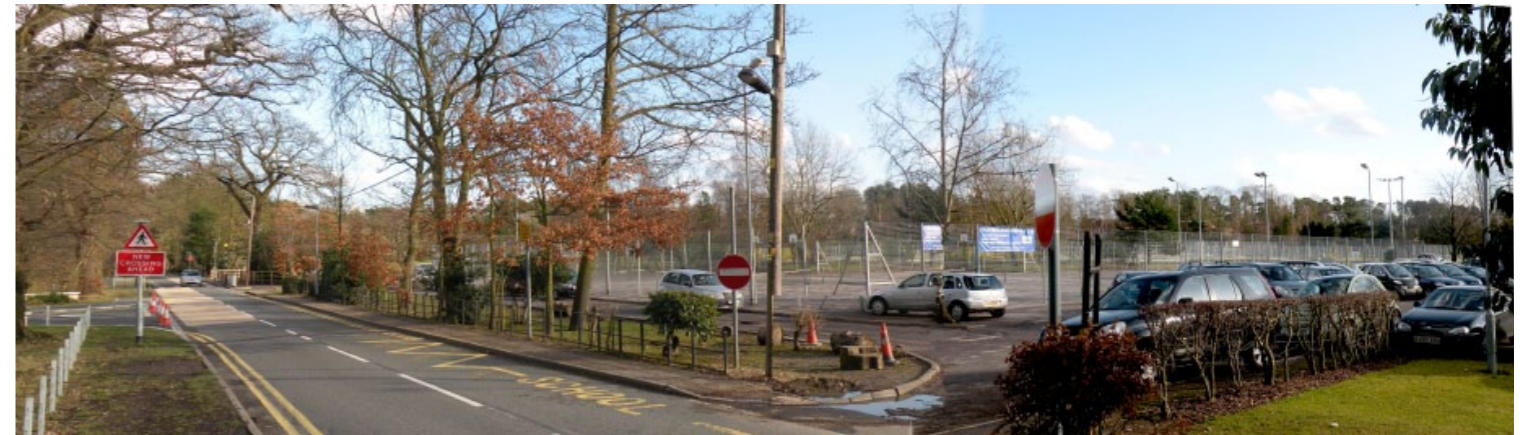
View of the site looking west from Charters Road
